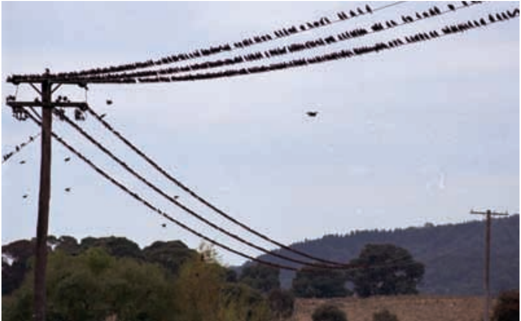
Figure 2.8: Starlings perching on powerlines. Photo: B. Lukins.
